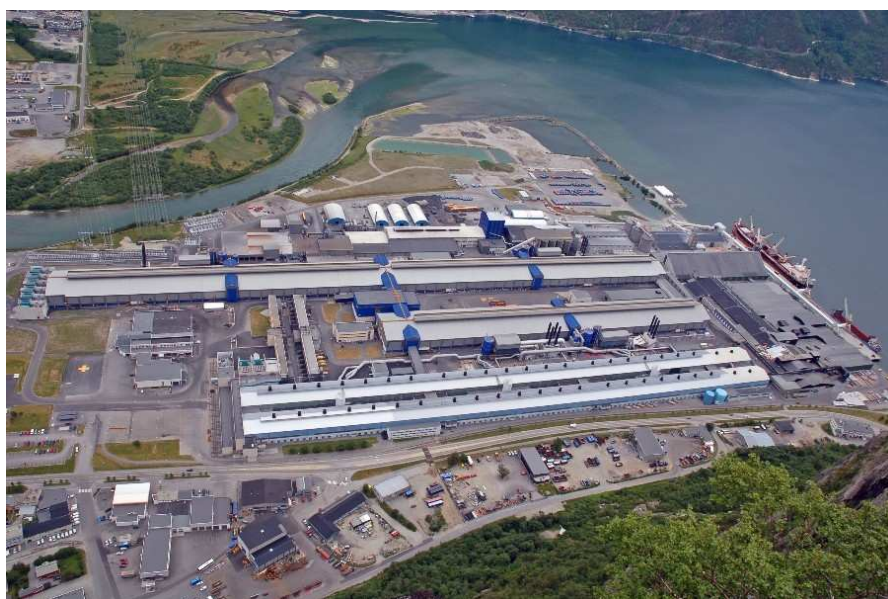
The Sunndalsøra plant, Norway modern (partly) Söderberg-based aluminium smelter: Class 4 low emitter
